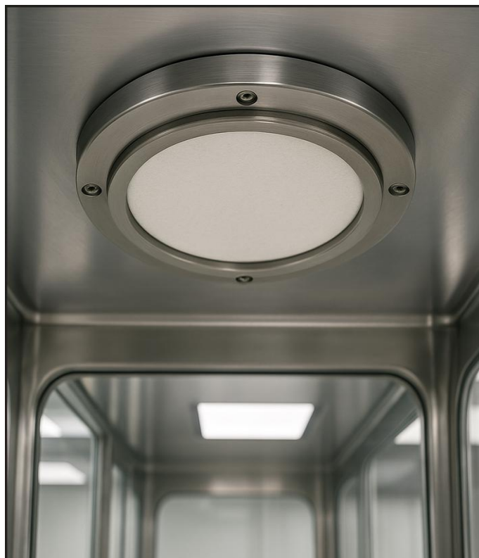
Figure 4: Refurbished CG membrane post-reconditioning. White upper and lower sheets (PETP -SEFARE PETEX 07.44/25) remain intact, ensuring airflow diffusion and structural support.
