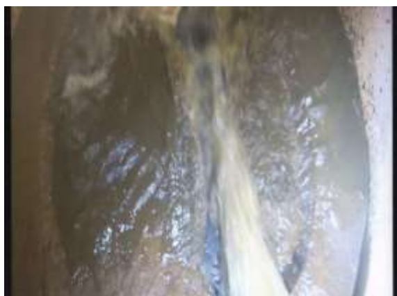
Figure 3: Sludge from WTP
